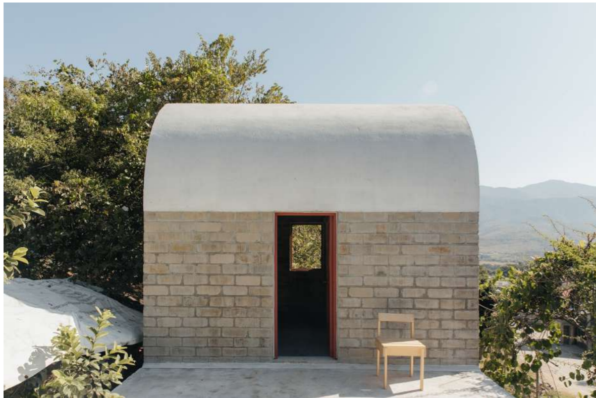
Roof with the additional terrace
